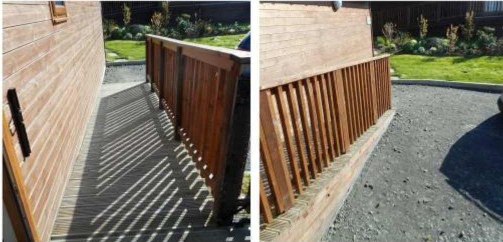
Tawny Lodge Ramp from Parking to Decking
