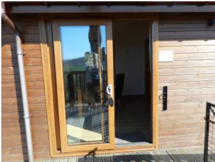
Tawny Lodge First Set of Patio Doors
