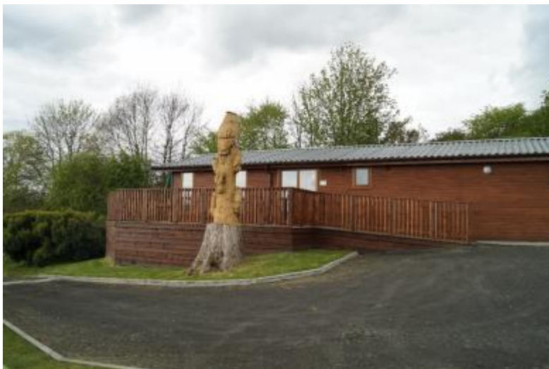
Parking Available to the front of Tawny Lodge
