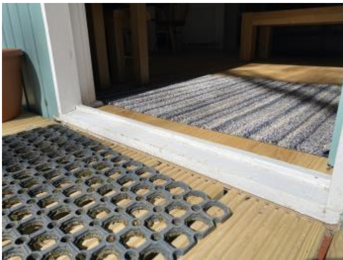
Step down to decking from lodge front door
