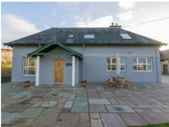
Level patio area leading to Chauffeurs Cottage entrance
